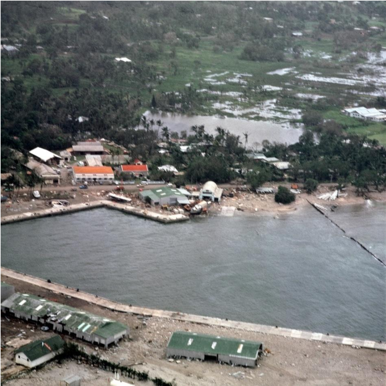
Figure 3.1: Post TC Sally (1987) Damage at Avatiu Harbour (Image: Don Dorrell)
