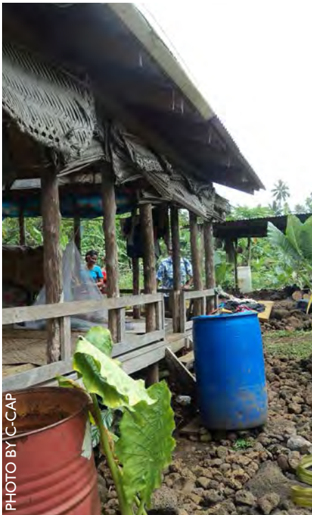
ABOVE: An existing household rainwater collection system in Sapapalii, Samoa, which will be replaced with a new collection and tank system through C-CAP.
