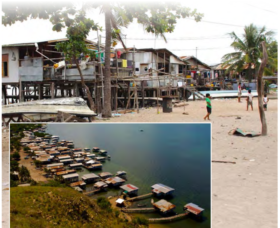
ABOVE and INSET: Buildings in Pari village which feature timber stilts and corrugated iron roofing are commonly built over seawater. Photos by C-CAP.
