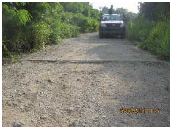
Figure 37. Horizontal scour checks
