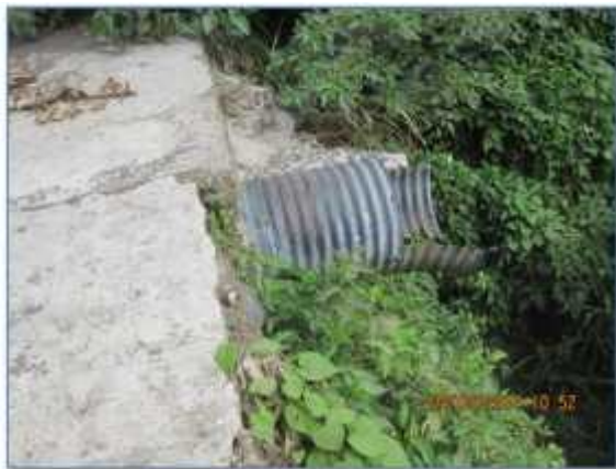
Figure 32. Cross drainage poorly maintained
