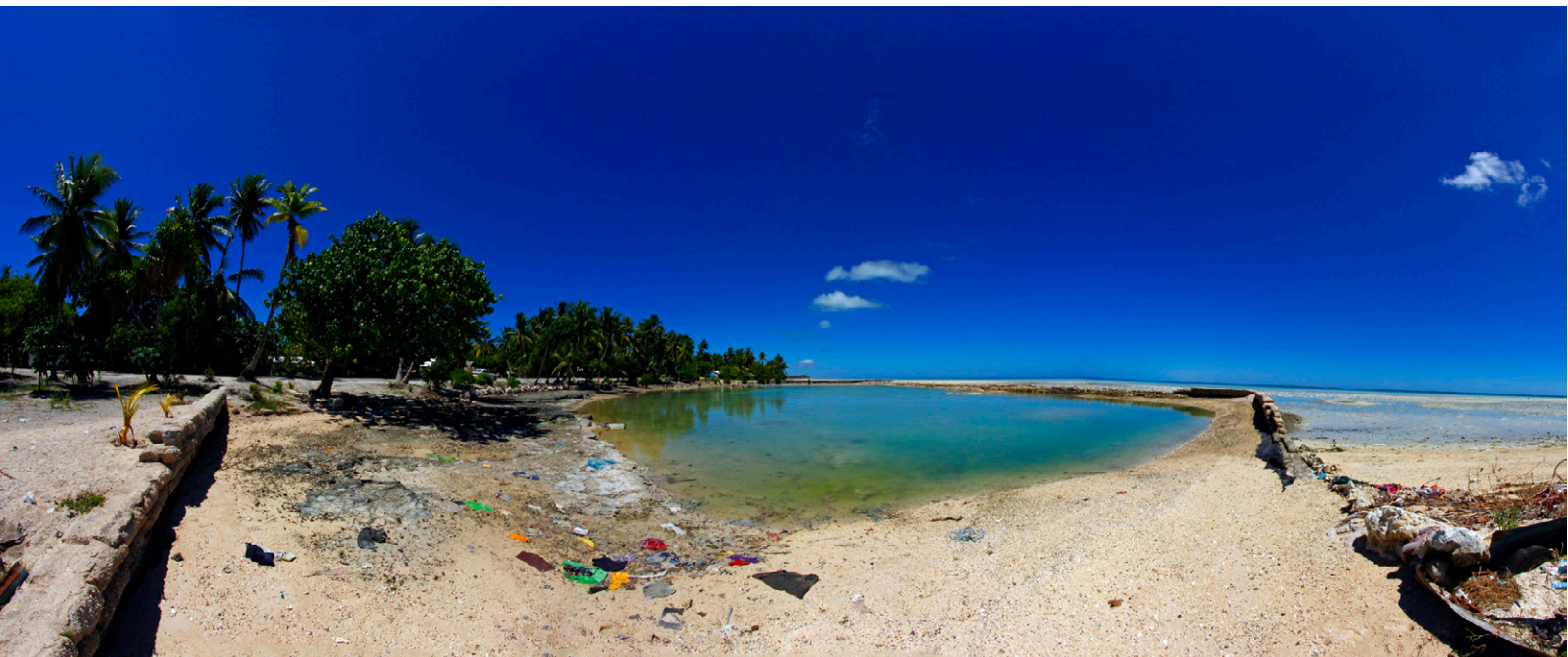
ABOVE: Coastal scene in Kiribati showing placement of stone walls and other materials to reclaim land and prevent future coastline erosion. Photo by C-CAP.
