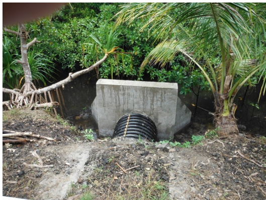
36 inches culvert headwalls
