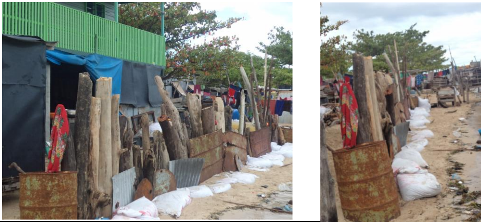
Fig. 6: Temporary sea walls (wood, drum, etc) erected on the island to prevent storm surge or rising sea level.
