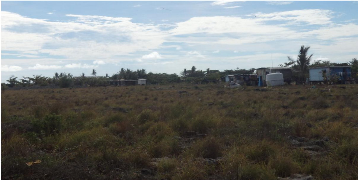
Fig. 7: A few houses being built on rocky surfaces as shown here, and the area in the foreground is covered with limestone rocks.
