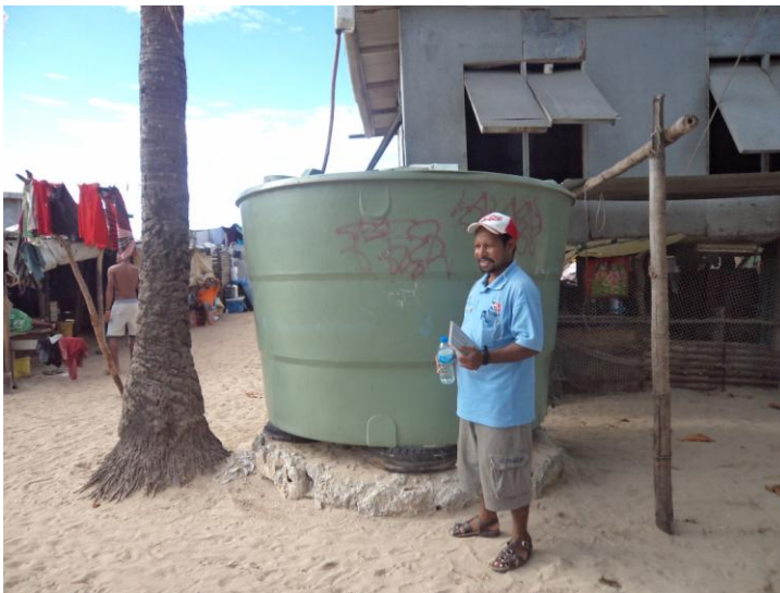
Fig. 5: Water tanks given by European Union, no proper foundation to support tank as this picture shows.
