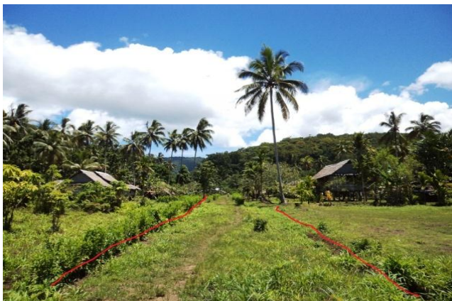
Figure 9: Drains (indicated by red lines) like these were dug in the village to not only divert but to accommodate flood and rising sea waters as well (photo by P. Ramohia).
