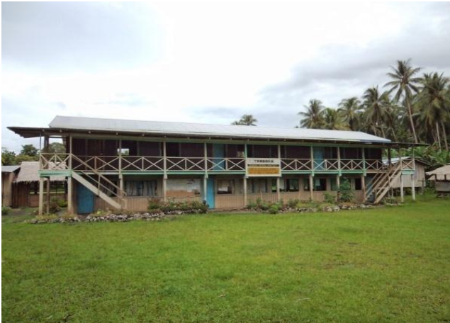
Figure 2: The Tamboko primary school building funded by the Australian government (photo by P. Ramohia).
