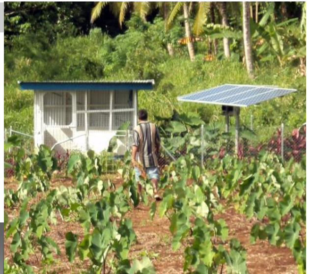
Photo: Solar power in Tonga
